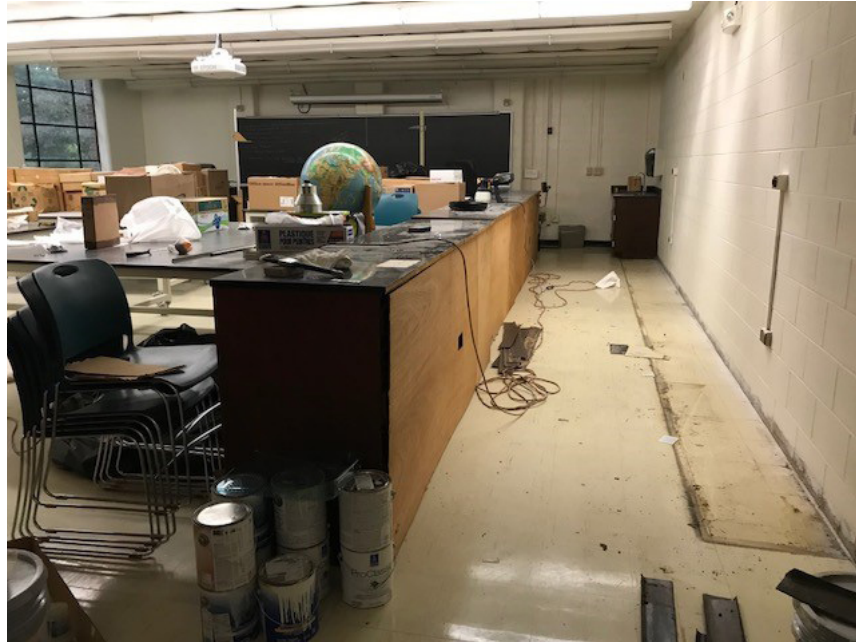
Lafferty 108 during the renovations
