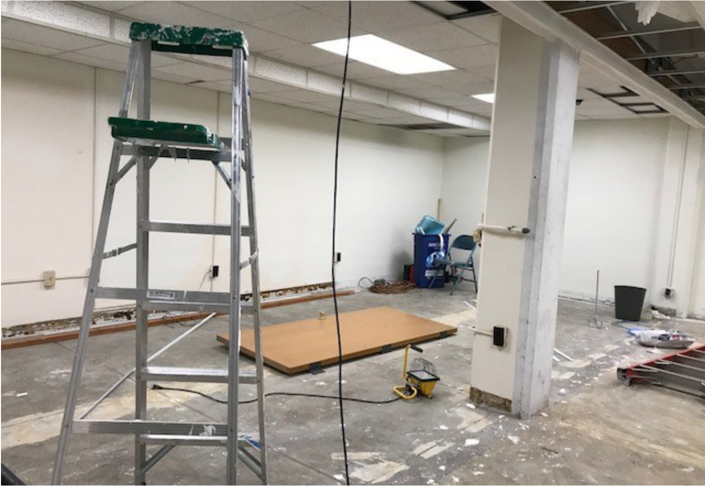
Lafferty 101 during the renovations
